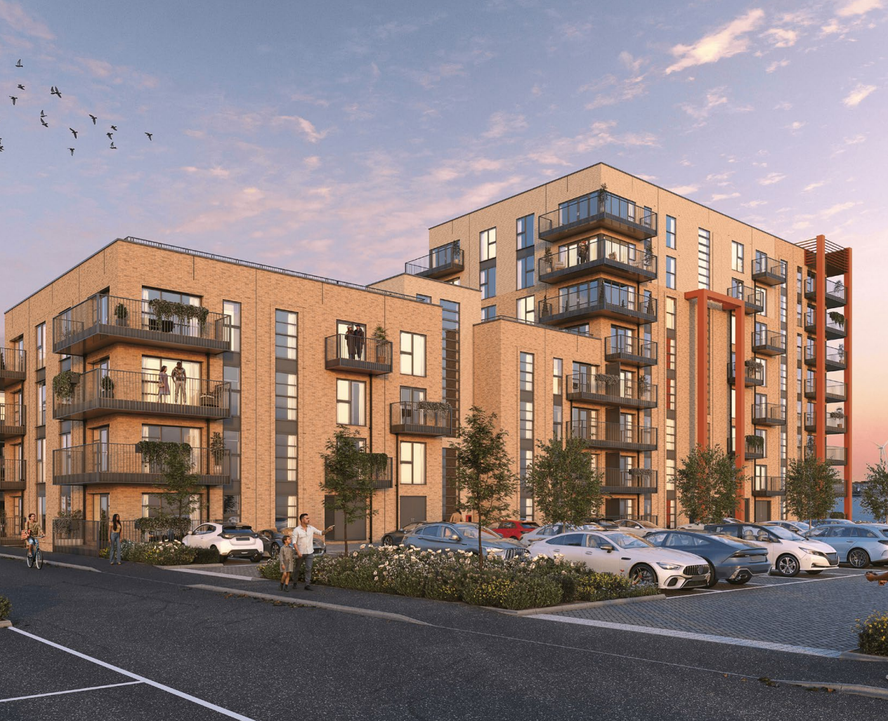
Faraday heights sits proudly at 4 stories as an shared owners only apartment in its entirety, adjacent the 6 storey waterfront building.
